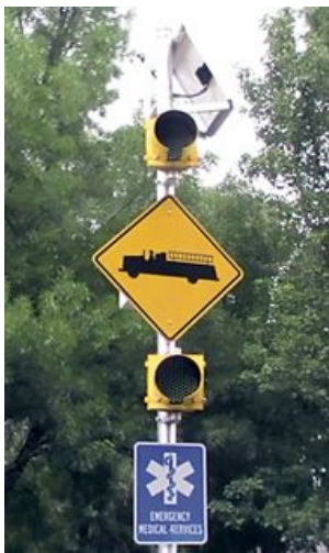
Typical solar powered EVCS.
